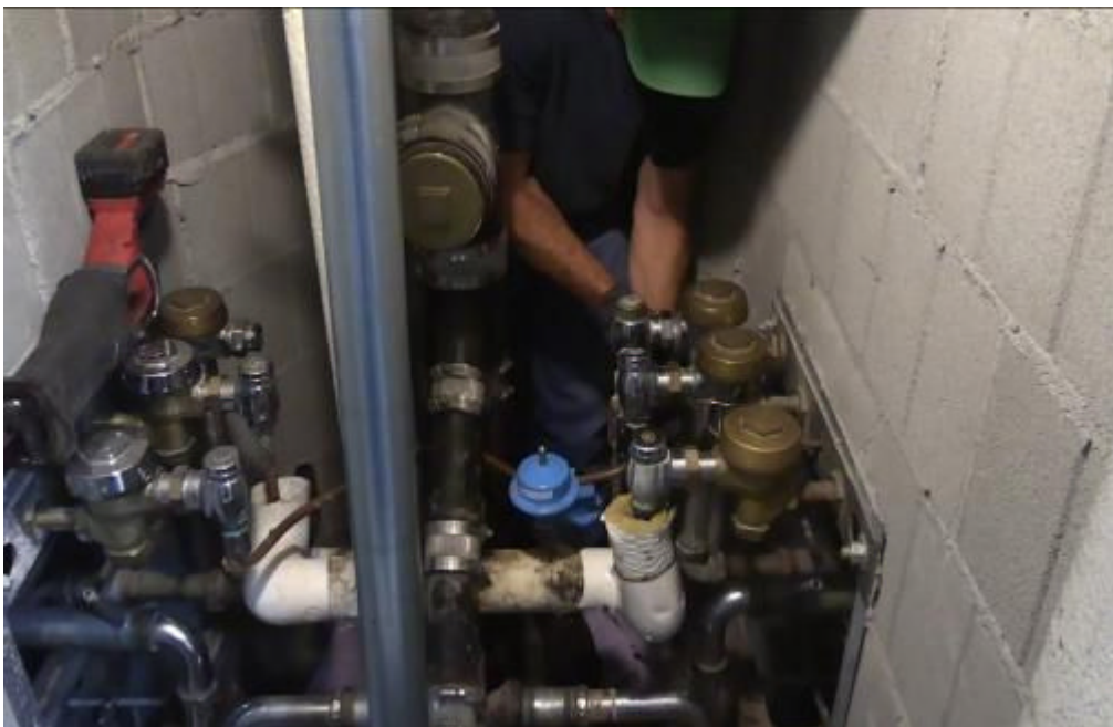
Plumbers often work in confined spaces such as the plumbing chase, show here. A chase is the space between each cell that houses plumbing, electrical and HVAC components.
